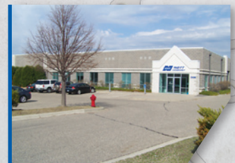
Burnsville Manufacturing Burnsville, MN
